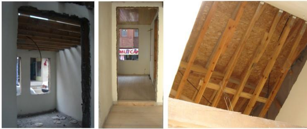
Figure 22. Reconstruction of the buildings with traditional techniques and roof details
