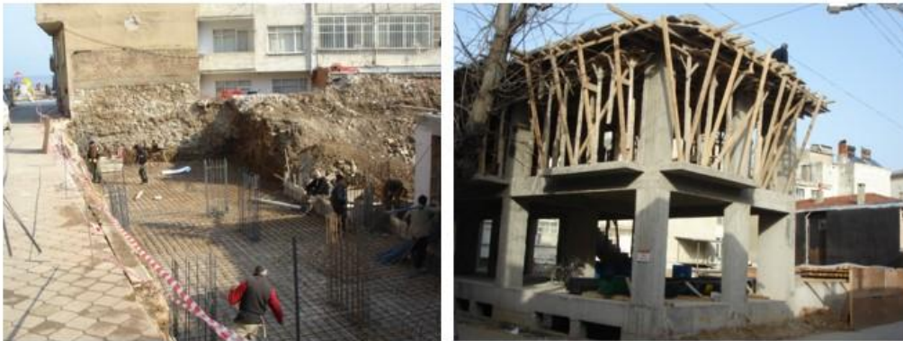
Figure 19. Construction of parcels numbers 11 and 12
