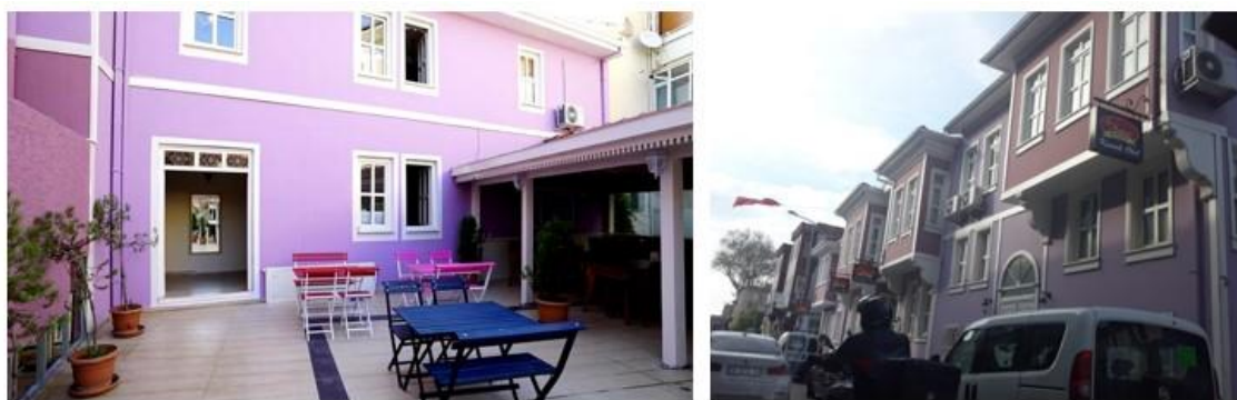
Figure 26. Post-restoration of the buildings, a view from the courtyard
