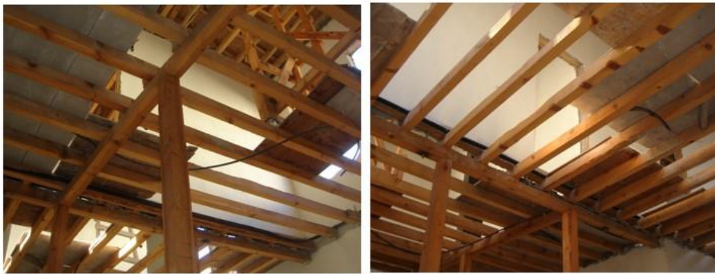
Figure 23. Construction of floor covering
